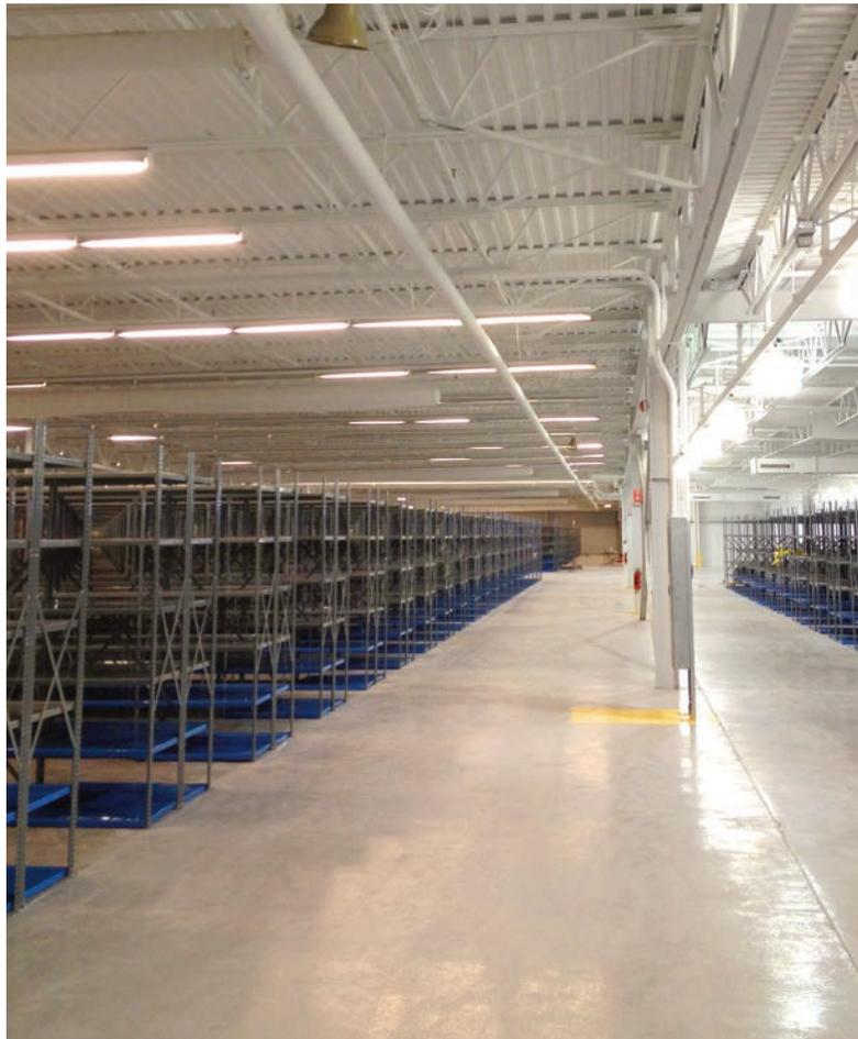
This picture shows the WPSS Deluxe shelving designed to support the conveyor system from the top of the sections prior to the installation of the conveyor system.
