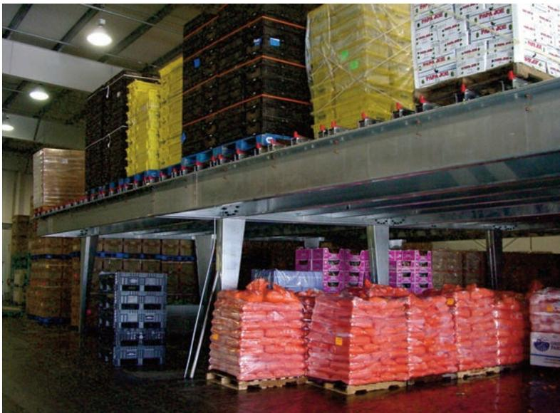
Working under a tight three-week production deadline, a 14,000 sq. ft. custom wide-span platform (mezzanine) was designed and built over the facility's existing dock area with compliance to code and clearance requirements. The platform (mezzanine) span had to correlate with the building's column span of 44' and handle a load of 150 Psi.
